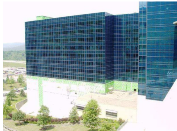
Figure 2 - South Elevation Photo Courtesy of Jim Boje, PE (Wendel)
